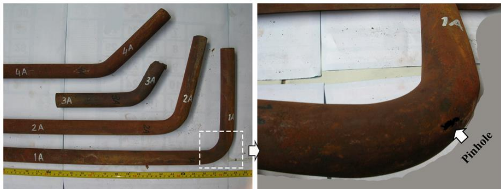
Figure 2. Four elbow tubes (1A to 4A) cut away from the low pressure evaporator evaporator outlet header, where one of the elbow tubes (1A) shows a pinhole on the outer side of the elbow curvature
