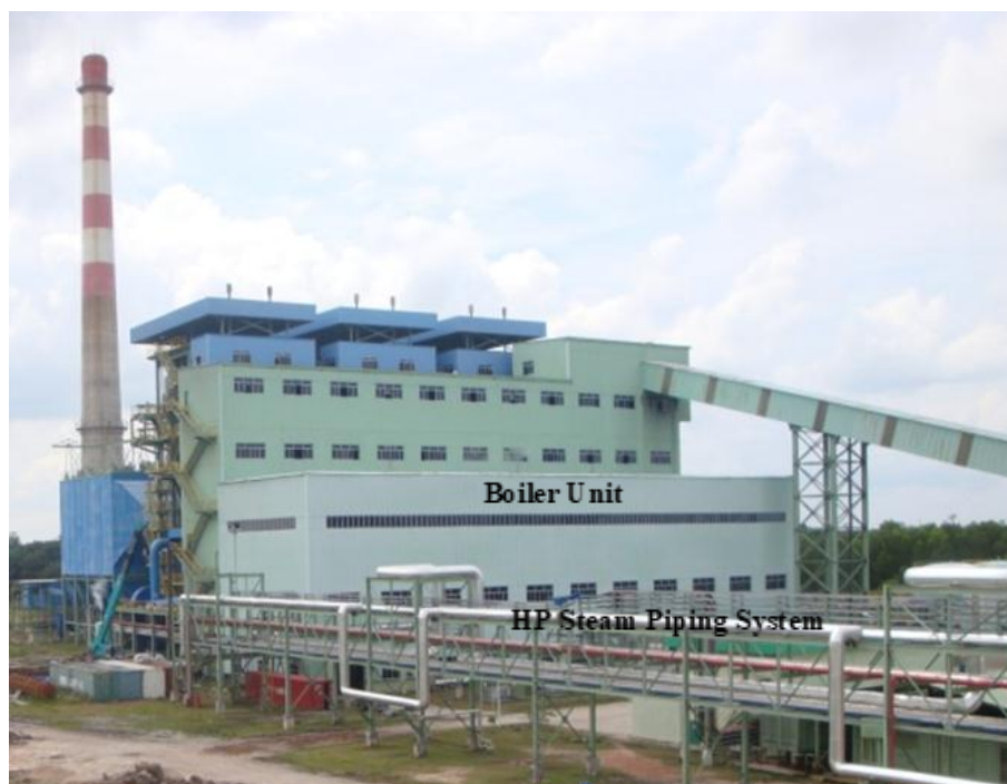
Figure 1. A newly built boiler construction and its corresponding HP steam piping system, connected to a palm oil processing unit at location approximately on the right hand side (not seen)
