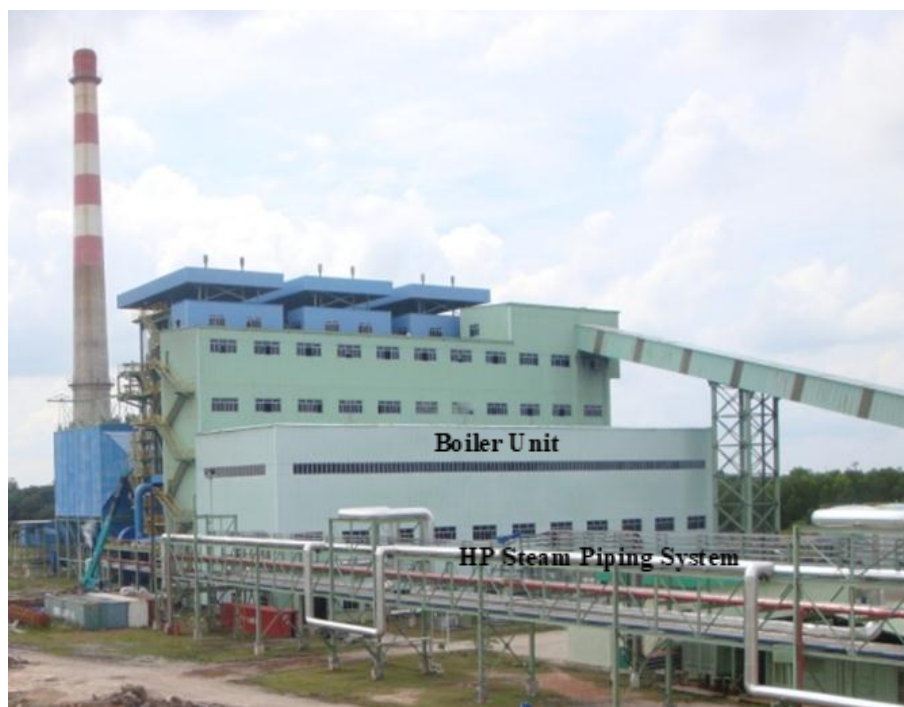
Figure 1. A newly built boiler construction and its corresponding HP steam piping system, connected to a palm oil processing unit at location approximately on the right hand side (not seen)
